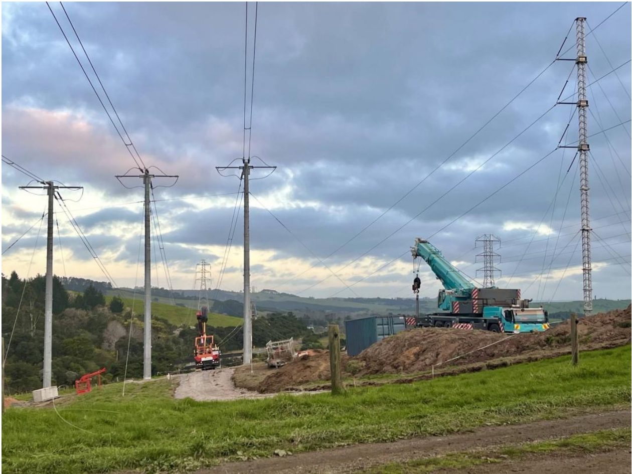
Figure 9. Temporary 220 kV circuit structures
