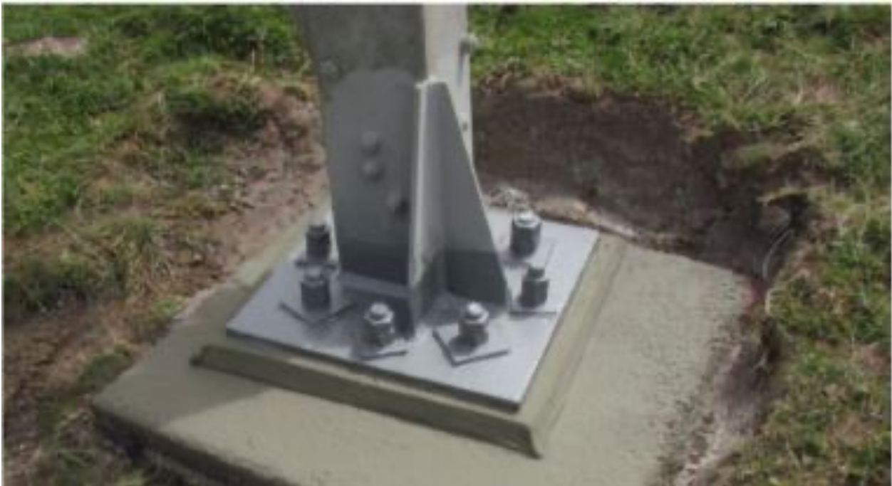
Figure 6: Refurbished tower foundation
