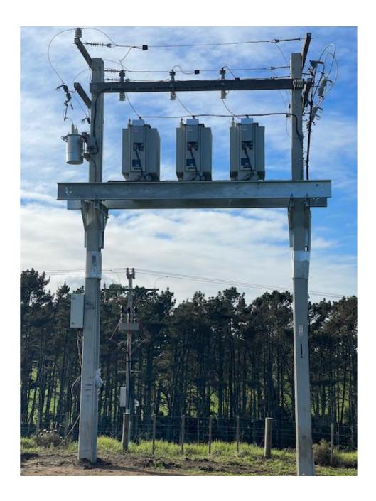
An additional benefit of our STATCOM unit is its ability to smooth out faults in the grid. It does this by rapidly switching between absorbing and producing reactive power to either increase or decrease the voltage of each line individually. This effect increases the reliability of our connection with the grid by preventing unnecessary trips (a historical problem of ours).
