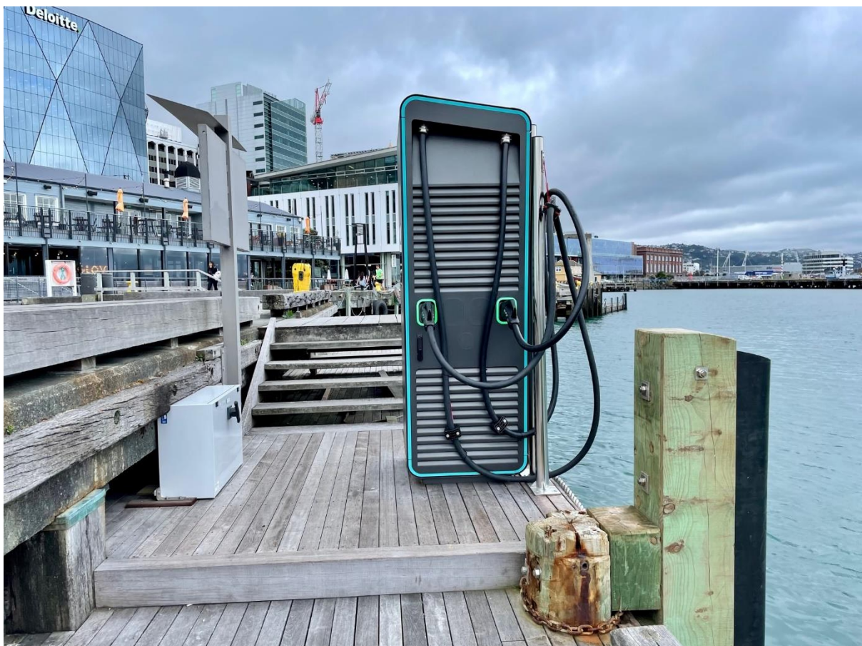
Photo: Charging infrastructure for the East by West electric ferry in Wellington, photo © Elizabeth Yeaman 2022
